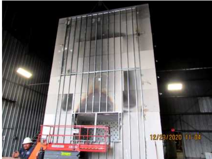
Photo No. 1 Installation of Metal Stud Frame Wall
