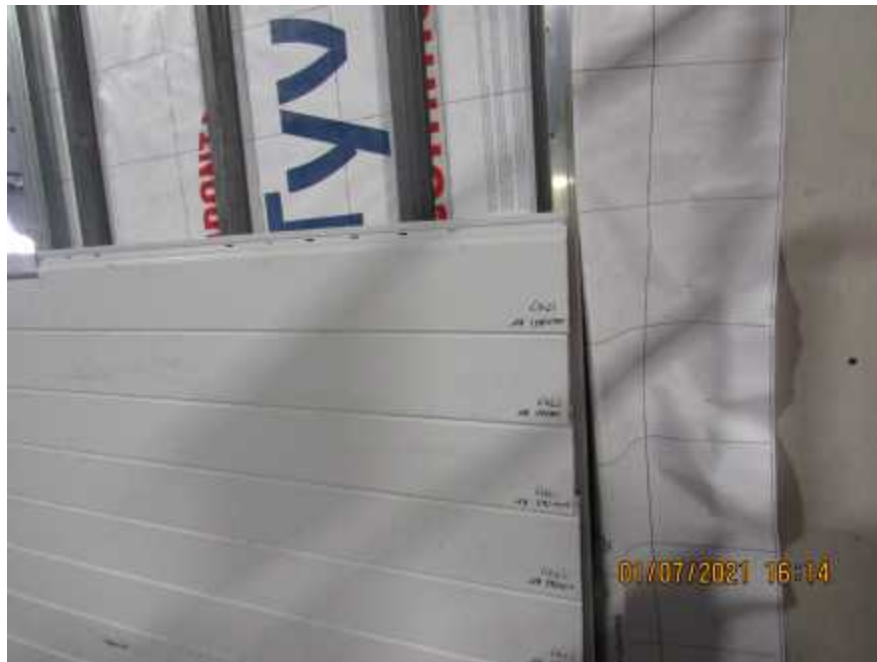
Photo No. 5 Installation of ChamClad PVC Siding
