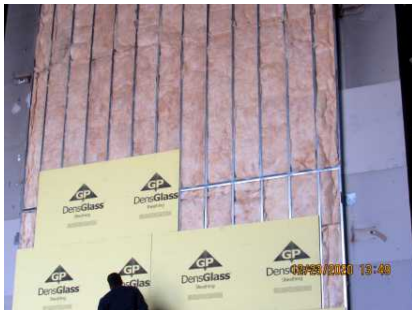
Photo No. 2 Exterior Sheathing and Stud Cavity Insulation Installation
