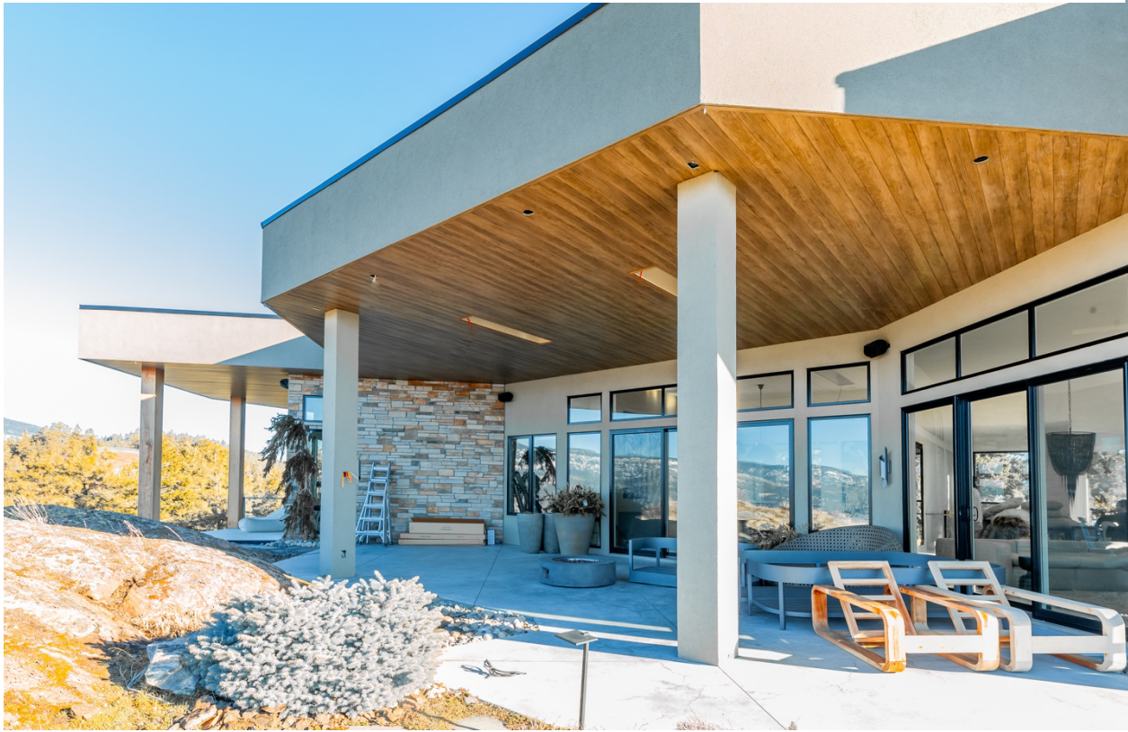
Soffit – Perpendicular to Building
