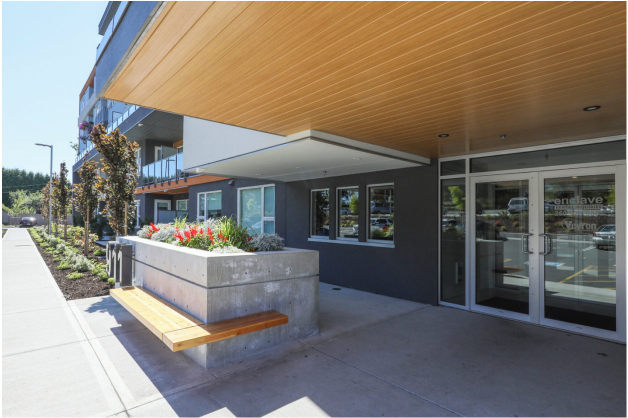
Soffit - Parallel to Building
