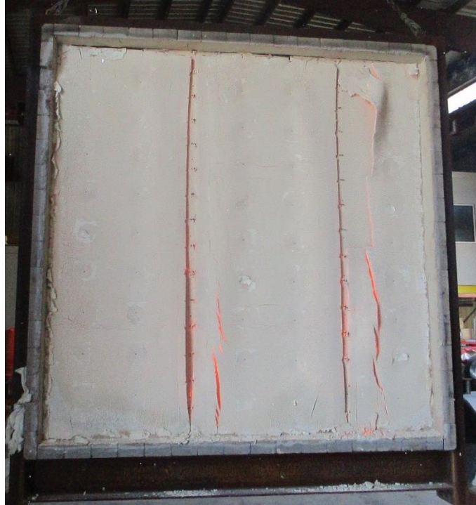
Photo No. 21 Interior Exposure - Exposed face – (Post-Fire Resistance Period)
