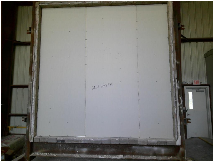
Photo No. 4 Completed base layer of GWB on unexposed face Interior Exposure
