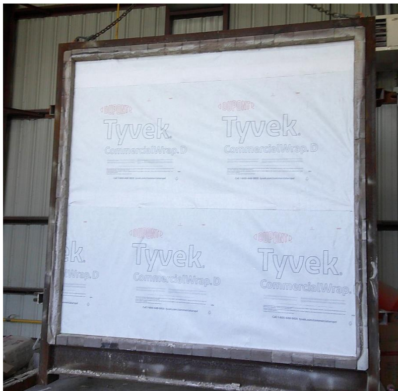
Photo No. 6 Completed installation of WRB on unexposed face Interior Exposure
