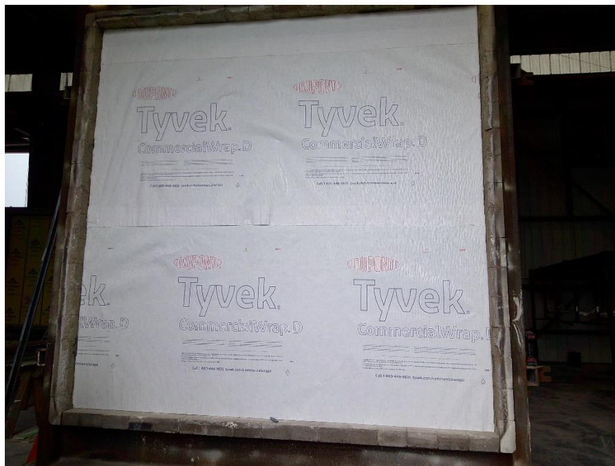
Photo No. 32 Completed installation of WRB on exposed face Exterior Exposure
