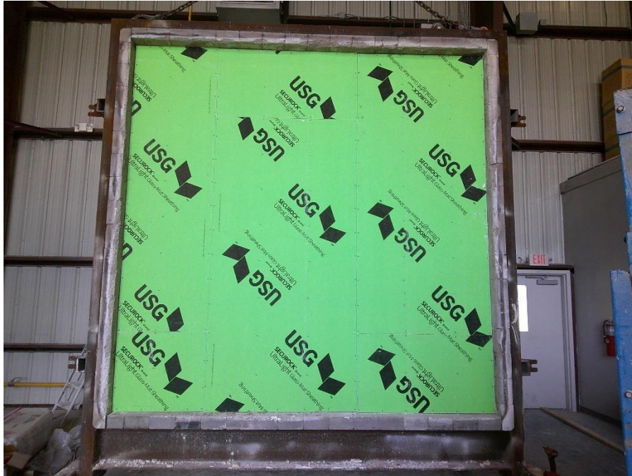
Photo No. 5 Completed face layer of Exterior GWB on unexposed face Interior Exposure
