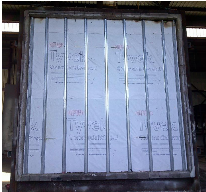
Photo No. 24 Interior Exposure - Char Extent of WRB – (Post-Mortem Observations)
