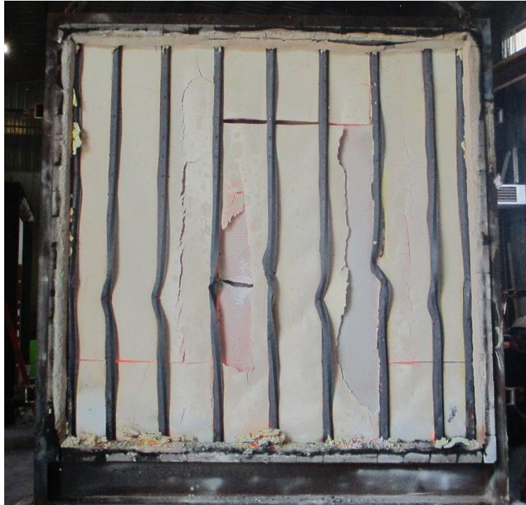
Photo No. 41 Exterior Exposure - Exposed face – (Post-Fire Resistance Period)
