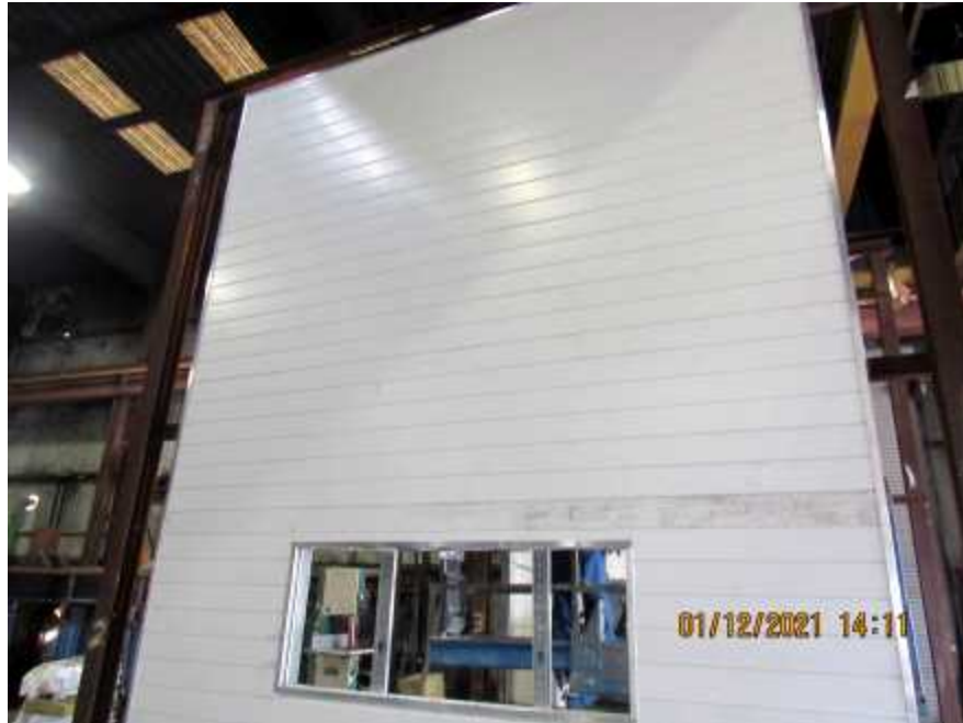
Photo No. 3 Finished View of PVC Cladding Installation
