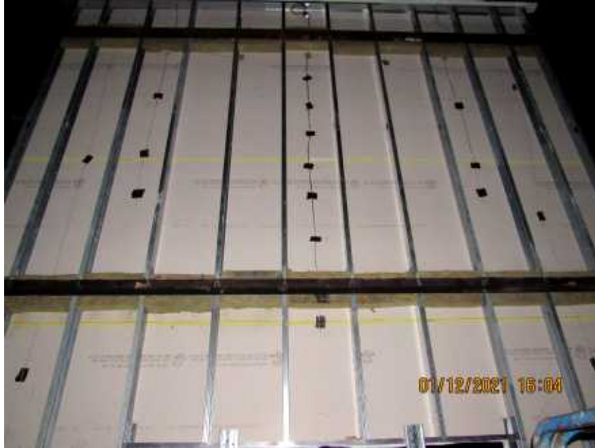
Photo No. 1 Rear-View of Wall, Prior to Insulation and Gypsum Installation
