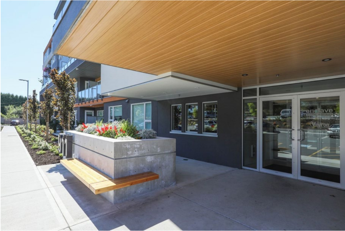
Traditional Soffit – Parallel to Building
