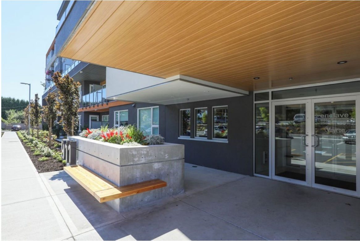
Traditional Soffit – Parallel to Building
